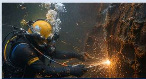
Underwater Cutting Operation
