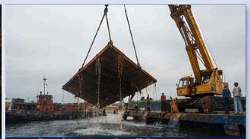
Breaking into Small Pieces within Lifting Capacity
