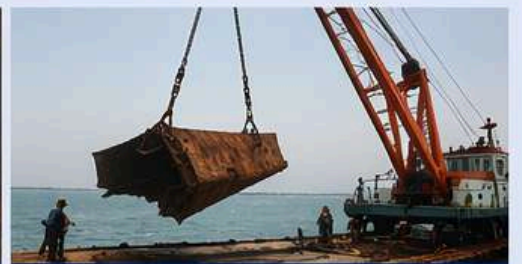
Retrieval of Cut Pieces to Surface
