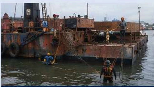
Underwater Inspection & Marking
